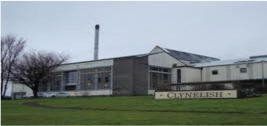
*Clynelish Distillery will see the installation of an additional mashtun, 10 new washbacks and six new copper stills. This adds to the 10 washbacks and six stills which the distillery currently has, and will effectively double the production capacity to nine million litres of alcohol per annum, whilst retaining the unique character and quality of the spirit.*
